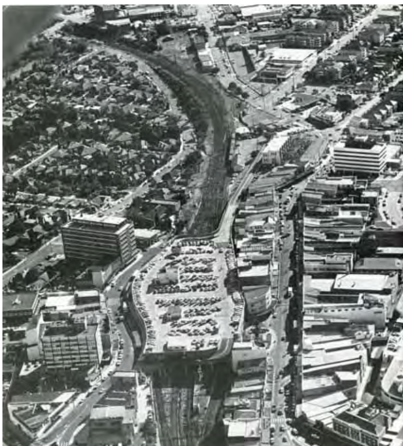
Figure 74: This aerial view of Hurstville shows the shopping centre of Forest Road on the right with the Supercentre straddling the railway line in the centre of the foreground. The Hurstville Story
