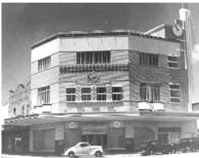
Figure 67: Electricity House still stands at 213 Forest Road Hurstville. Hurstville City Library Local Studies Collection
