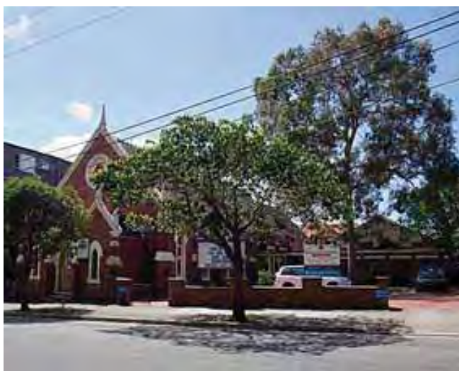
Figure 51: The Uniting Church, formerly the Methodist Church at The Avenue, Hurstville was built in 1903. It is home to a 1929 Whitehouse Organ which also survives. Photos Arthur Lee, October 2011 www.sydneyorgan.com/HurstvilleMeth.html
