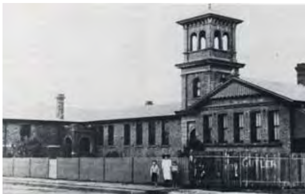
Figure 50: Hurstville Public School in about 1910 1913. The building with the tower was added in 1891. The Hurstville Story
