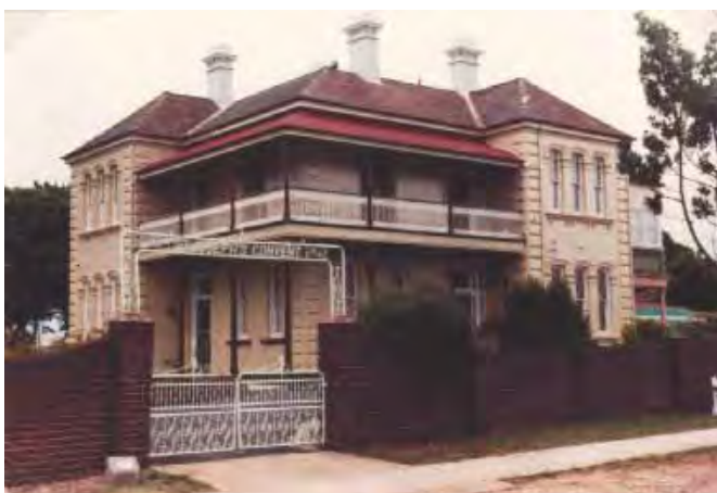
Figure 26: St Joseph's Convent at the corner of Forest Road and Penshurst Street was originally Rostrov, the home of John Sproule who built it in 1886. Sproule was a builder who built several homes in Penshurst, living in each one until the next was ready for him, before selling them to others. Hurstville City Library Local Studies Collection
