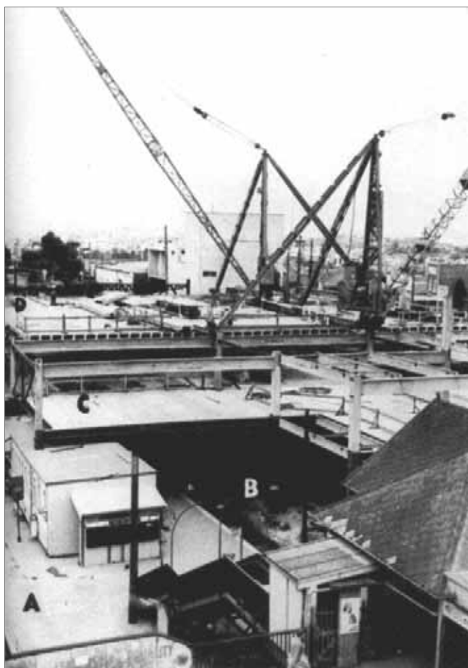
Figure 73: This image shows the progress on the construction of the new Hurstville Super Centre over the Railway Station in 1963. Bernard Sargeant, The History of Hurstville Council , 2
