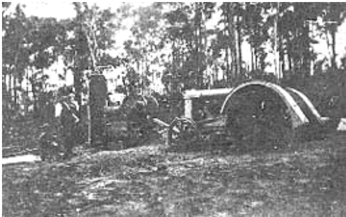
Figure 14: This image of the Lugarno stone quarry shows a stone cutting machine with a crane or pile driver behind it. Hurstville City Library Local Studies Collection
