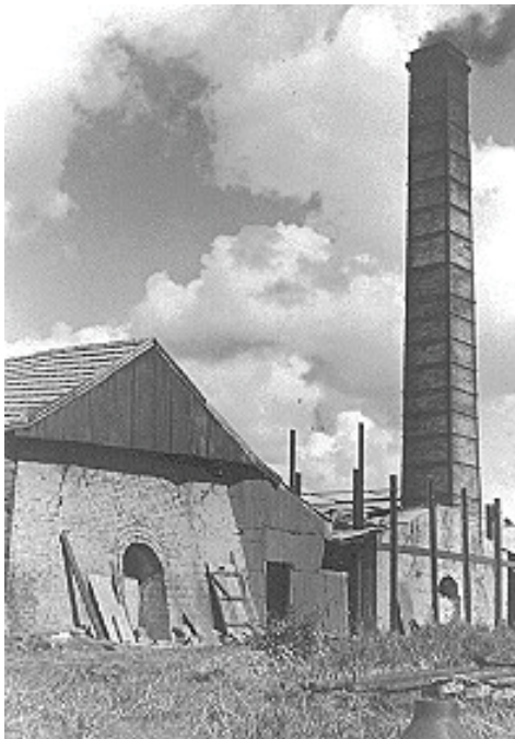
Figure 58: This image shows the two downdraught kilns ashman built c. 1918 20 as part of his extension of buildings and plant. Hurstville City Library Local Studies Collection
