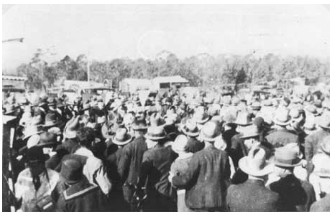
Figure 20: A large crowd assembled at Padstow to watch Premier Lang turn the first sod to begin construction of the East Hills Railway ceremony on 3 September 1927. Hurstville City Library Local Studies Collection
