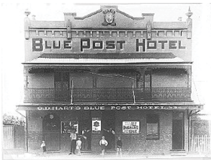
Figure 35: By 1925 the Blue Post Inn had been greatly modified into a two storey building in a late nineteenth century style. Hurstville City Library Local Studies Collection
