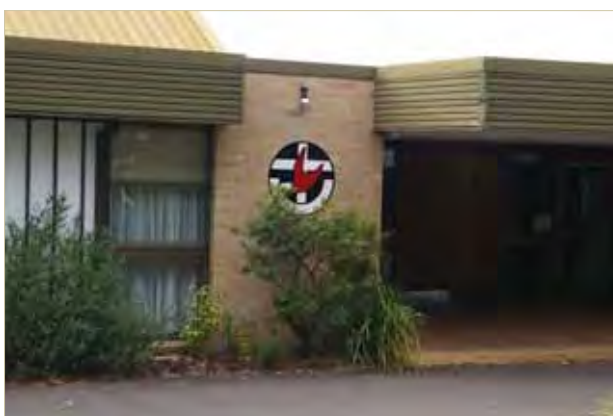
Figure 58: The Lugarno Peakhurst Uniting Church is located at 909 911 Forest Road Lugarno. Picture from www.lpuc.org.au
